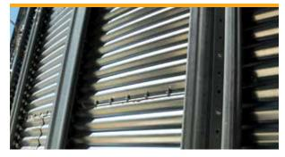
GSI bins are constructed using the hightensile steel (rated up to 70,000 psi) for higher capacity and superior protection.
