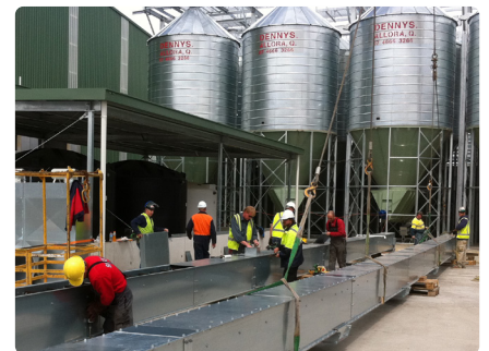
SKIOLD & VMS specialize in installation with trained technicians, installers and supervisors
